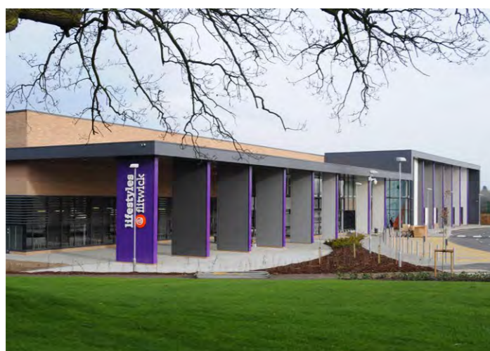
Figure 241: Flitwick Leisure centre
